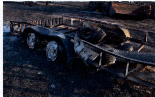
Damages sustained to trailers and equipment
