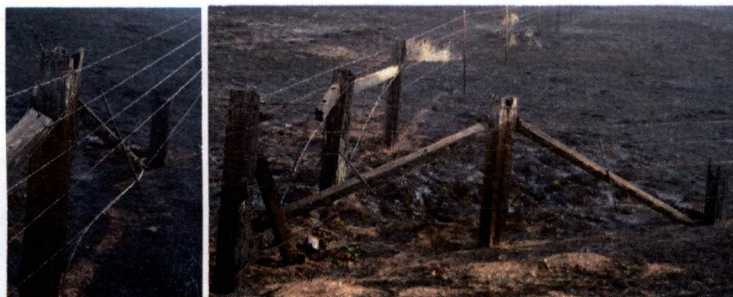
Numerous miles of Panhandle fences were destroyed in the wildfires
